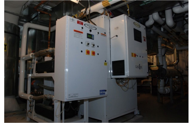
The test unit that captures anesthetic gases at Grand River Hospital, nicknamed Igor.
